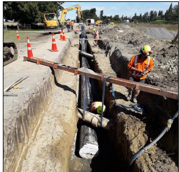
Crossing existing 300mm AC pipe
