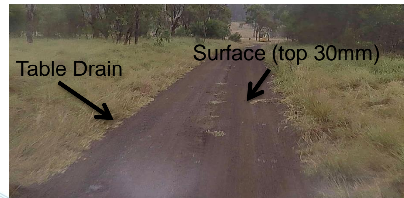
Figure 2. Formed Road (No Gravel)
