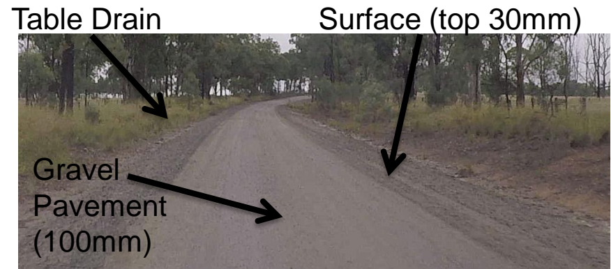
Figure 1. Formed and Gavelled Road
