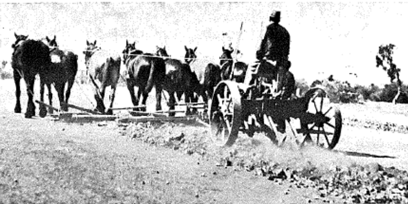
Early 1920s—A horse-drawn scarifier being used to rip up the old road surface in preparation for resheeting.
