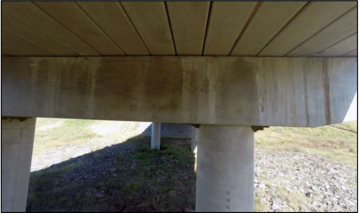
Figure 5: Underside of Bridge
