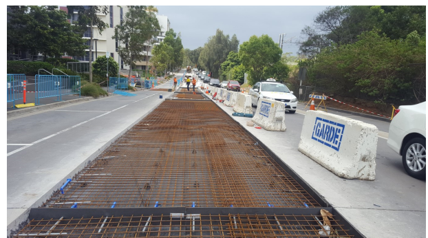
Figure 3: Full Slab Pavement Restoration Walker Street, Rhodes
