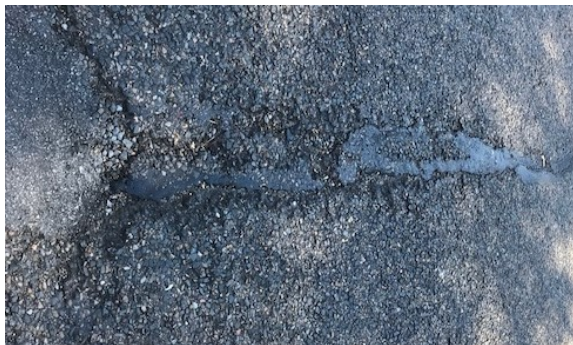
Figure 5: Reflected crack in Asphalt Overlay. Lyons Road West, Five Dock
