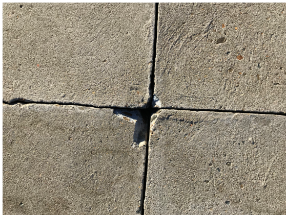
Figure 11: Clovelly Promenades slab joints showing little surface erosion after 15 years of service.
