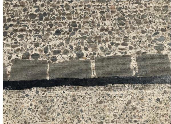
Figure 6: Trachyte used to protect the edge of the 1920's concrete at intersections. Note the larger aggregate of the 1920's concrete compared to the smaller sized aggregate possibly laid in the 1930's or 1940's. Pavement was planed in 2018 by NSW Roads and Maritime Services to reduce road noise and improve the ride. Lyons Road at Gipps Street, Drummoyne.
