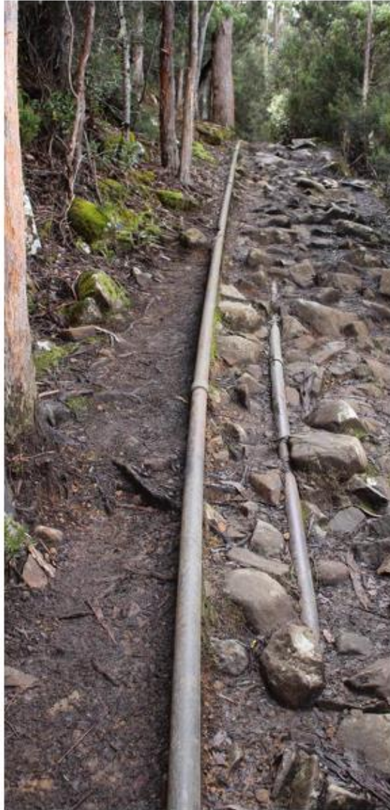
Figure 36: Mock-up of repair works along section with steep grade, water pipe and conduit
