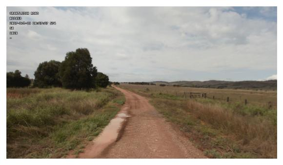
So using the same RACAS system this measurement is made every two years (depending on significant rain events, then it is done annually) to determine councils future re-sheeting and gravel patching programs for roads that are under the set service level by roads hierarchy.
