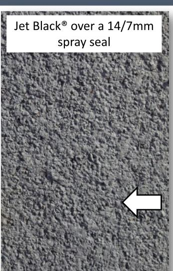
Picture taken from RAAF Base Curtin extremely oxidised surface treated with JetBlack to delay an expensive asphalt overlay
