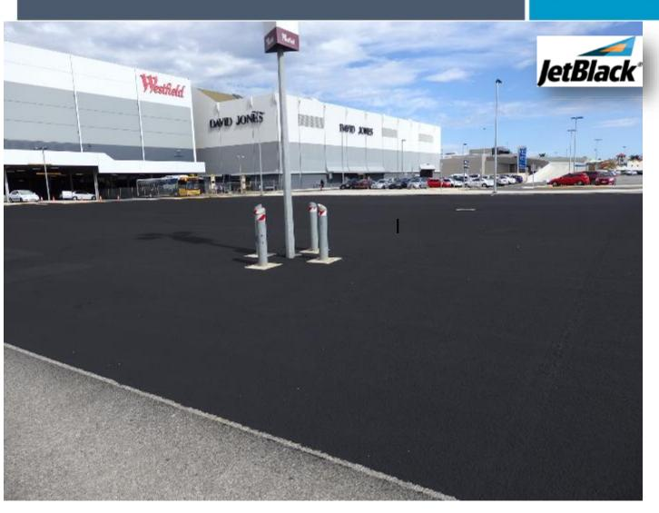
2015 treatment of asphalt car park that had patches placed throughout, Jet Black selected to prevent water penetrating the pavement and giving an aesthetically upgrade to a tired old pavement.
