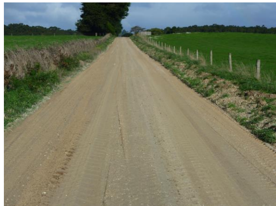
Resheeted Unsealed Road
