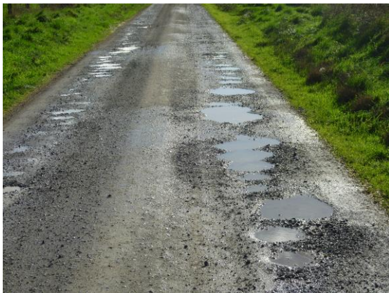
Unsealed Road prior to Resheeting
