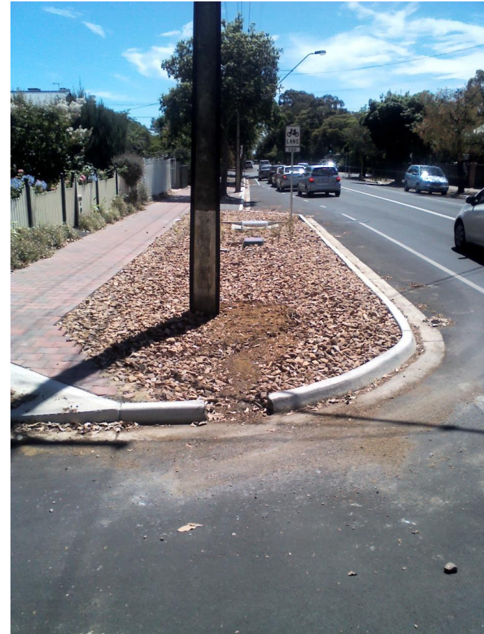
Bioretention in Wattle Street, Unley
