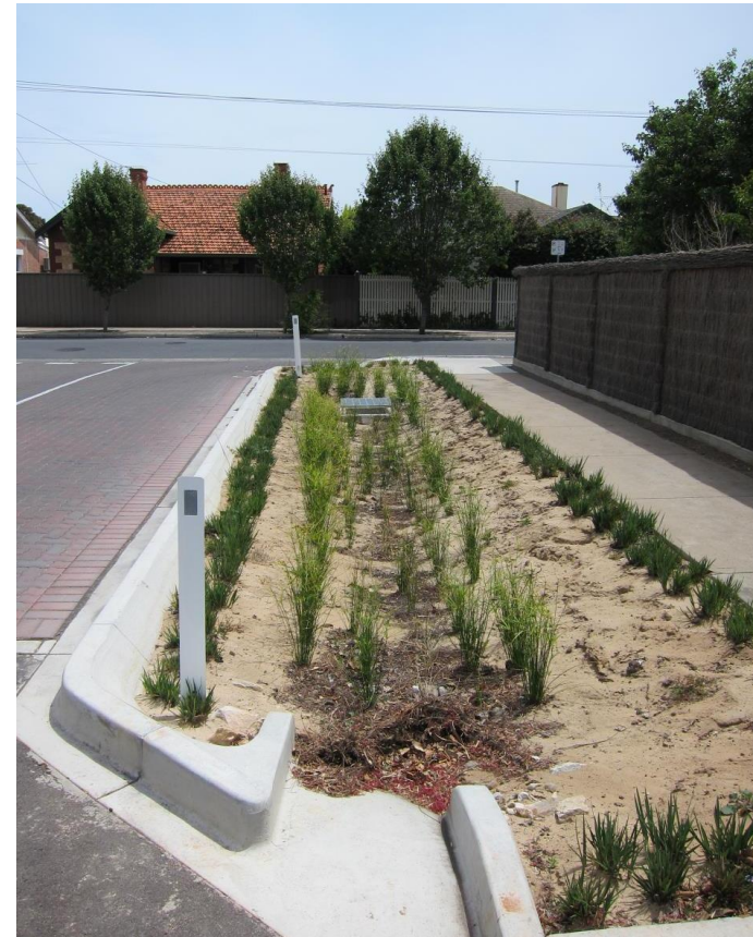
Bioretention basin, Mile End, City of West Torrens
