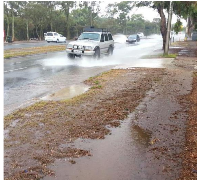
Minor system overflow, Para Hills
