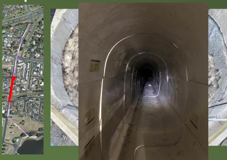
Pit 4 Cover removed for access 2.4 m dia depth 20 m **Tunnel Preparation GFRP Section** lowered into tunnel Assembly of liner Grouting liner in place Inside the liner Cost \$1.3m \$8700 per lineal metre
