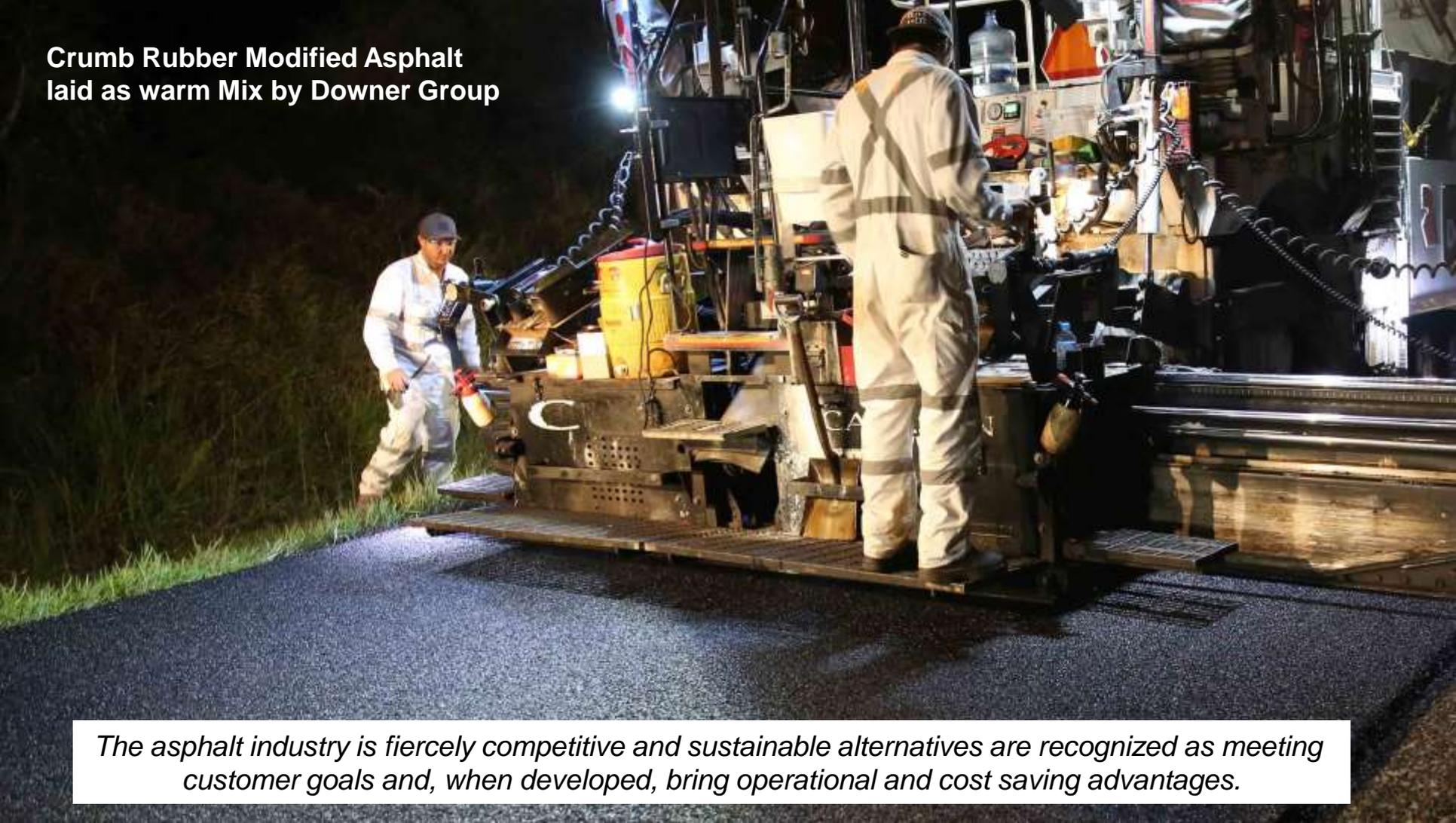
**Crumb Rubber Modified Asphalt
