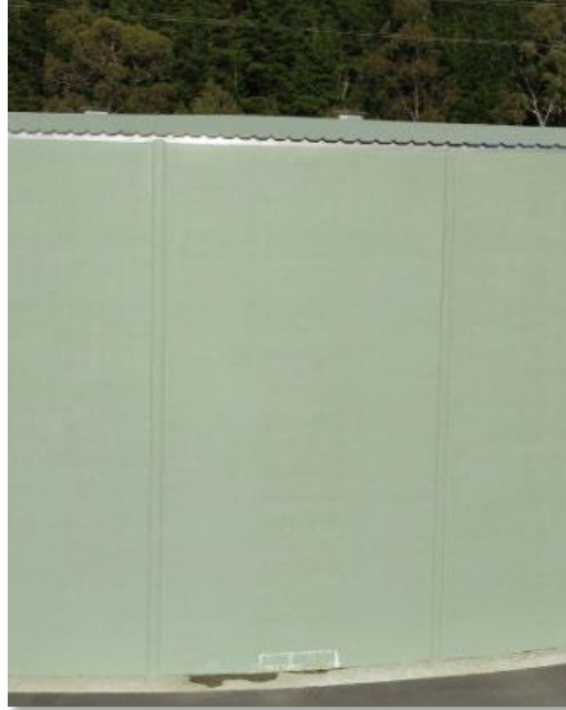
Post-tensioned panel construction reservoir showing signs of leakage
