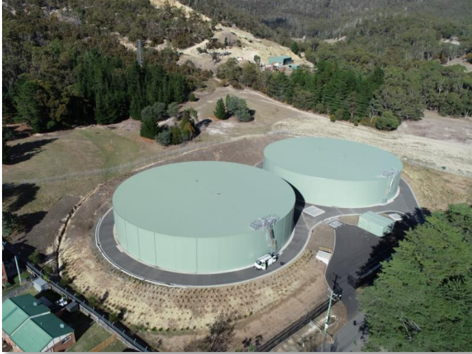
Post-tensioned panel construction reservoir showing signs of leakage
