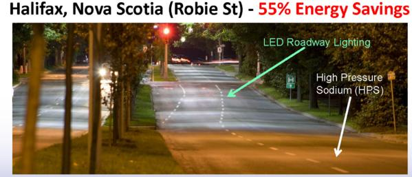
196 Watts HPS - 150W Bulb 88 Watts Satellite™ 96 LED-280mA
