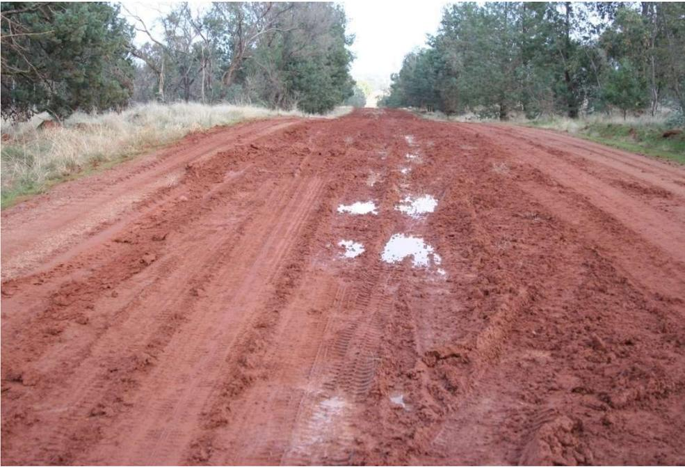
A non-stabilised unsealed pavement after rain
