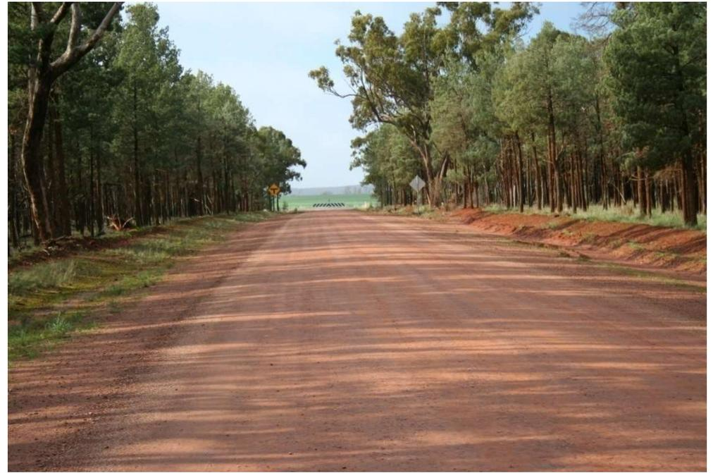
An adjacent lime-stabilised section after rain
