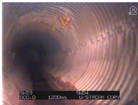
Figure 2: Reach 1 galvanised steel multi plate culverts, not rusted floor. 2
