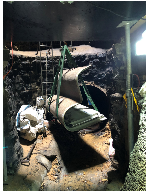
Figure 22: GFRP section being lowered into tunnel
