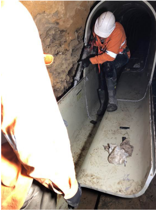
Figure 23: GFRP section being assembled
