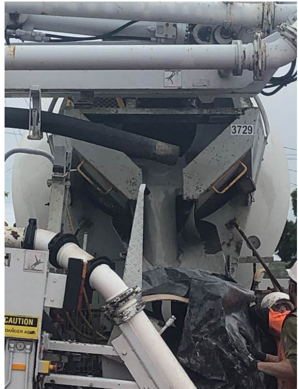
Figure 26: Grout 290 mm slump being pumped into tunnel
