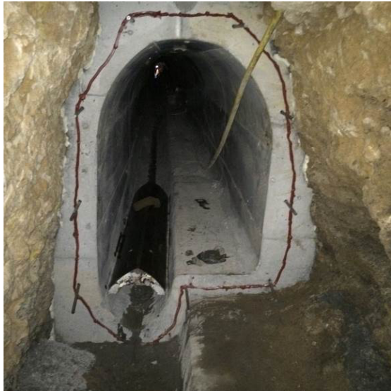
Figure 15: Tunneline after form stripped
