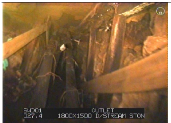
Figure 7: Downstream MH 5 collapsed timber shoring
