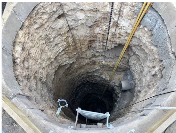
Figure 20: MH 4 20 meter deep, cover slab removed to provide access to tunnel
