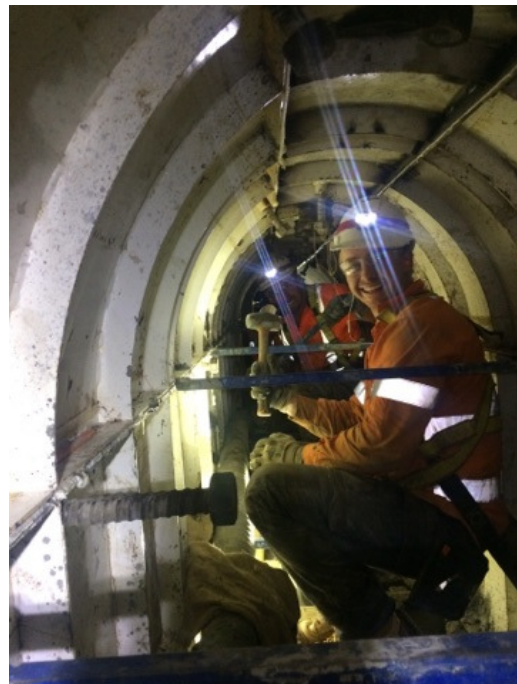
Figure 14: Tapping forms to remove air bubbles with hammer
