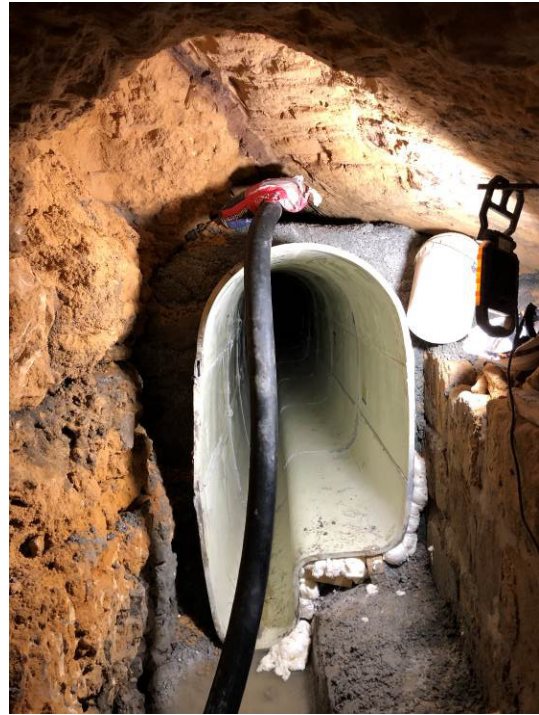
Figure 25: Grout hose in place
