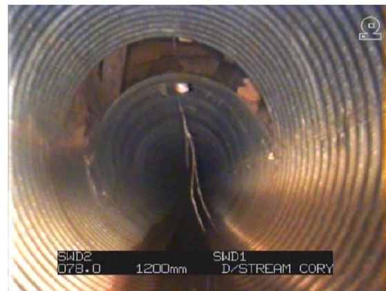
Figure 3: Dislodged section of multi-plate. 2
