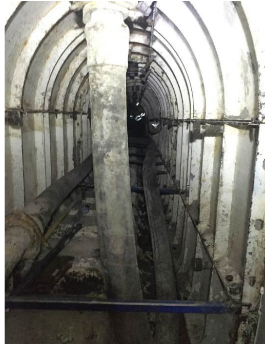
Figure 13: Tunneline form work with concrete hose in place
