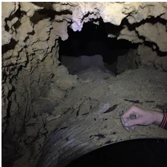
Figure 16: Entrance to void over multi-plate culvert
