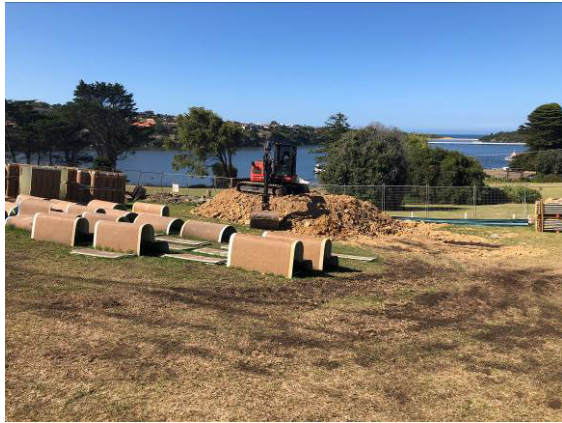
Figure 19: GFRP liner units awaiting installation
