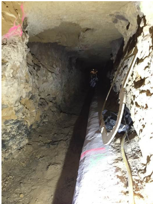
Figure 12: Tunnel excavated to size for Tunneline
