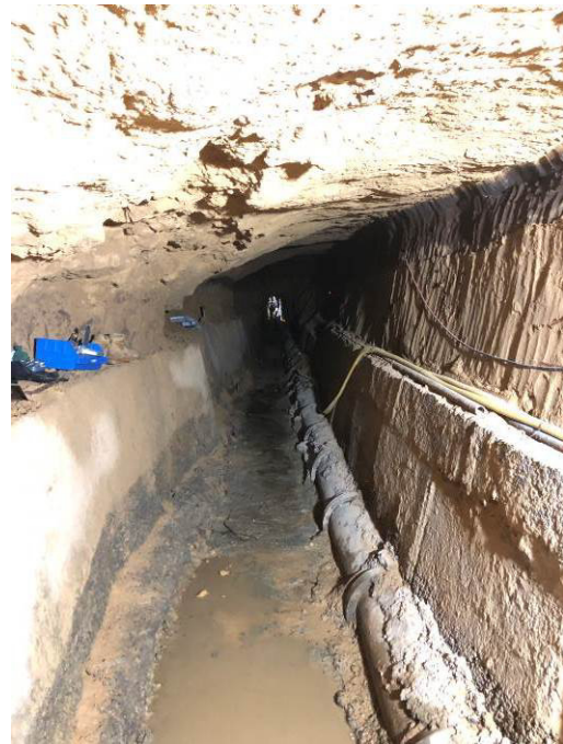
Figure 21: Tunnel downstream of MH 4, note sewer exposed
