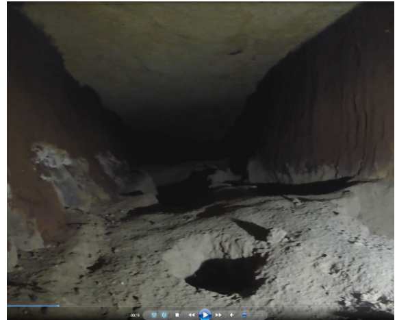
Figure 17: Void over multi-plate Culvert.
