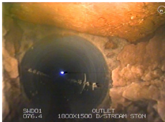
Figure 8: Figure 8 corrugated pipe downstream MH 5
