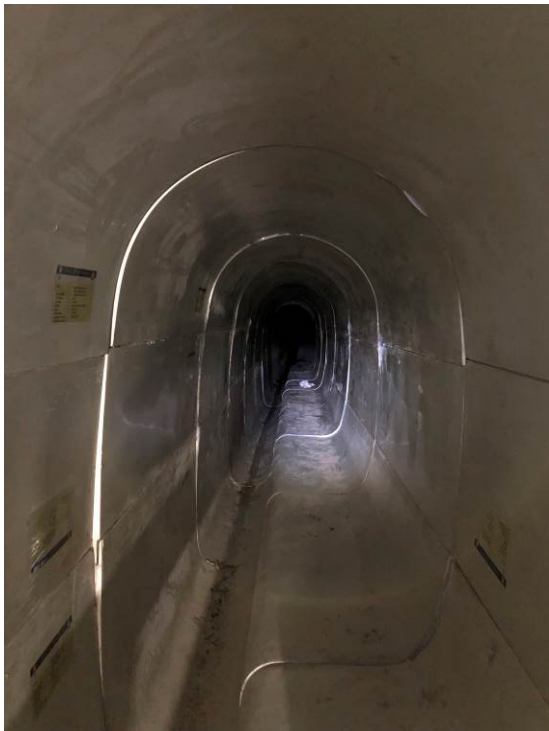
Figure 24: GFRP liner ready for grouting
