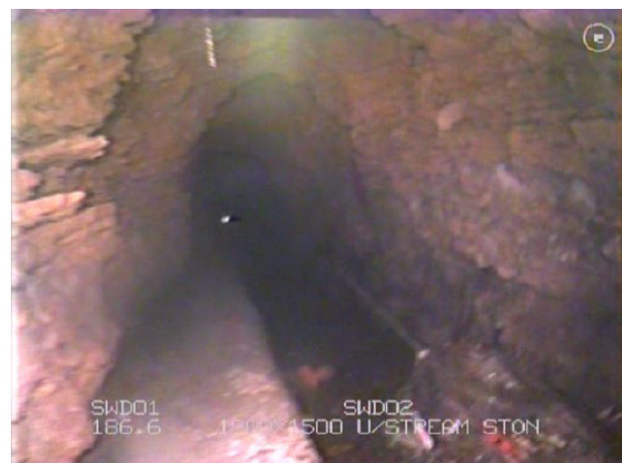
Figure 4: Tunnel between MH 4 and 5 looking upstream with sewer encasement on left 2
